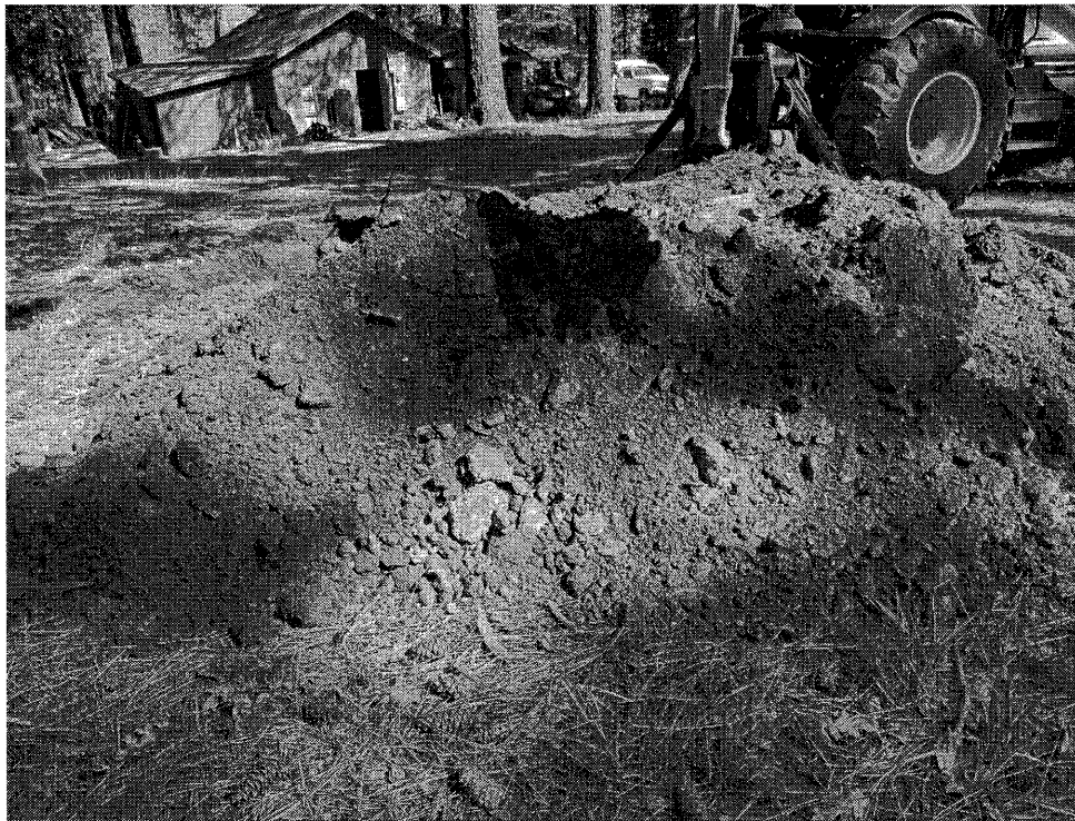
Photo No. 4 - Materials excavated from location TP2 including gravel from bedrock
