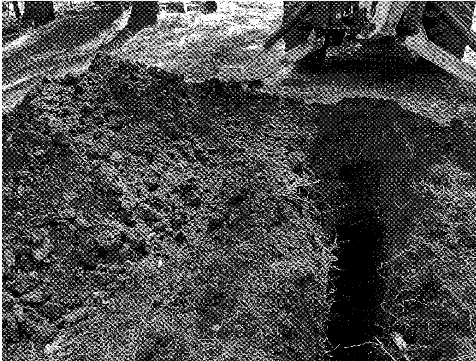
Photo No. 3 - Representative excavation characteristics at TP1
