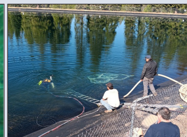
Debris Removal and Liner Inspection
