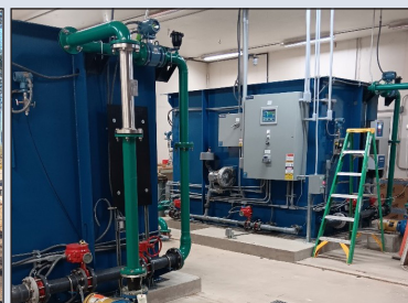
Installation of New Water Treatment Units
