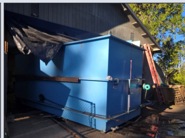
Removal of Old Water Treatment Units
