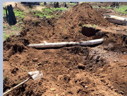
Leak repair along Eagle Ditch pipeline
