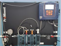
and installed by staff for New Prominent Chlorine Analyzer replaced older approximately \$12,000. failed and discontinued analyzer equipment
