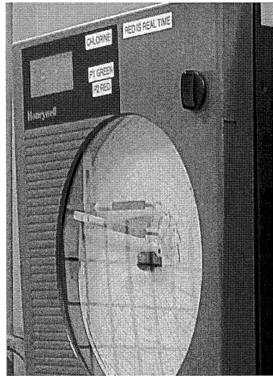
Closeup of Circle Chart for Chlorine Residual
