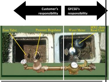
Shown above is a typical water meter box installation. Not every service looks like this, so please contact us if you need assistance! The "Gate Valve" is what customers should operate when winterizing their homes. Do not turn the valves on GFCSD's side of the meter. Only District staff is authorized to do so.
