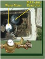
Above is a typical water meter box installation. Not every service looks like this, so please contact us if you need assistance. Do not turn the valves on GFCSD's side of the meter. Only District staff is authorized to do so.
