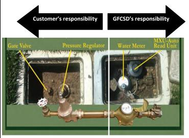
Above is a typical water meter box installation. Not every service looks like this, so please contact us if you need assistance. Do not turn the valves on GFCSD's side of the meter. Only District staff is authorized to do so.
